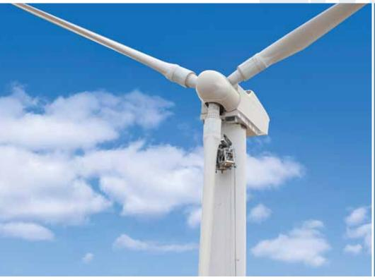
For blade inspection and repair operations, suspended platforms offer a safe, productive, and cost-effective alternative to cranes, groundbased lifts and rope access solutions.
