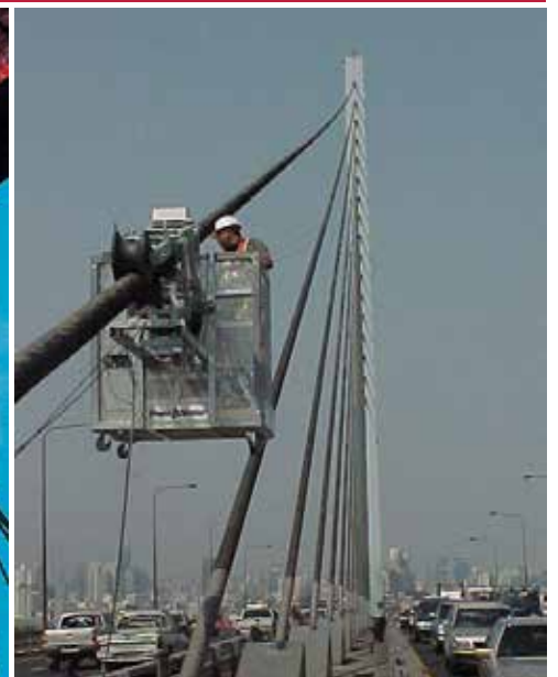
Rama Bridge Access - Thailand
